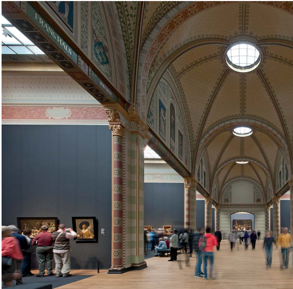
The laylights themselves are gently domed and above them are fluorescent lights, as well as a lot of vital technical equipment.
